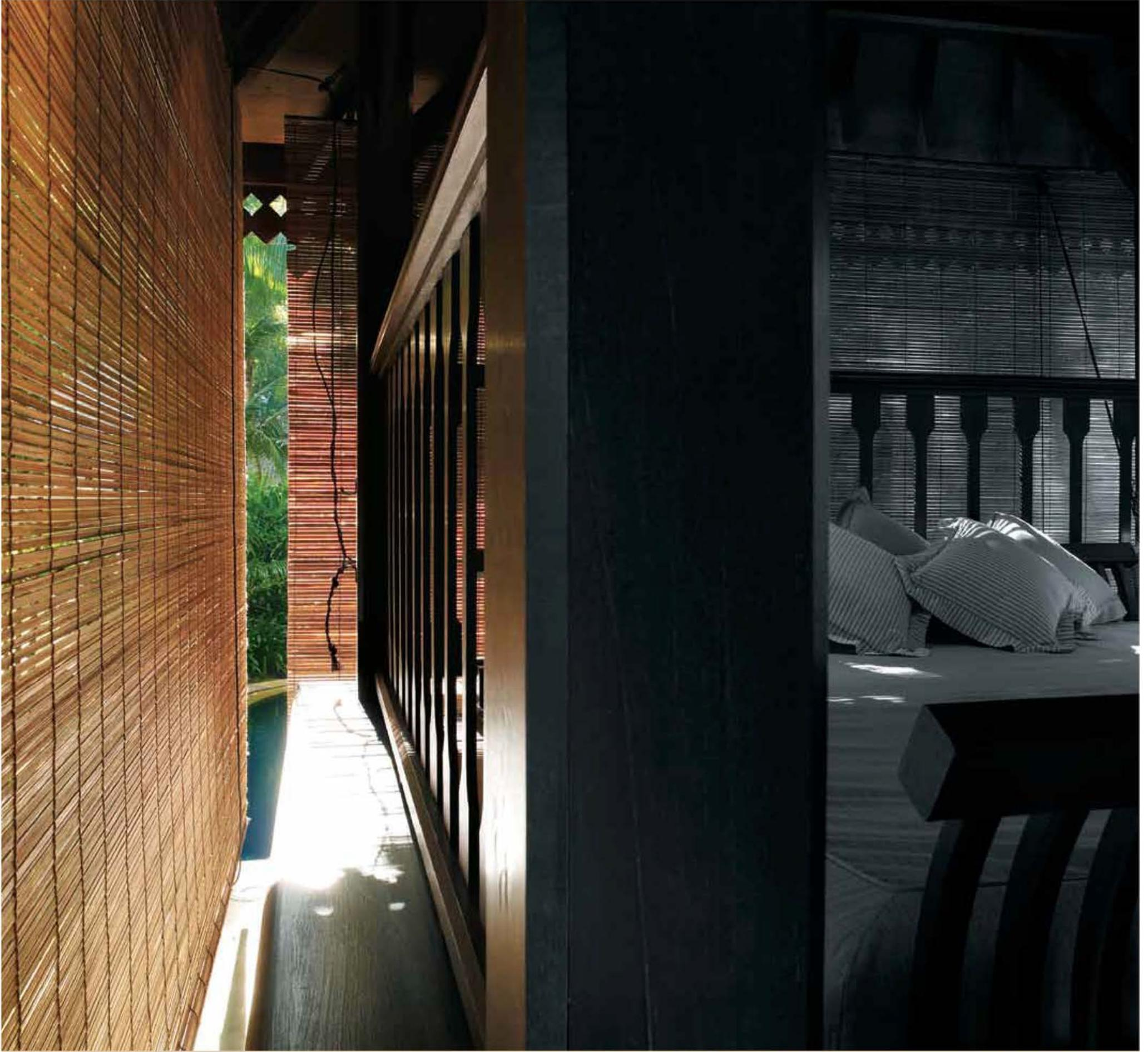
The resting pavilion utilises organic materials which can be locally grown like the fast-growing bamboo for its blinds. These blinds reduce solar gain while keeping the pavilion open to cooling sea breezes.
